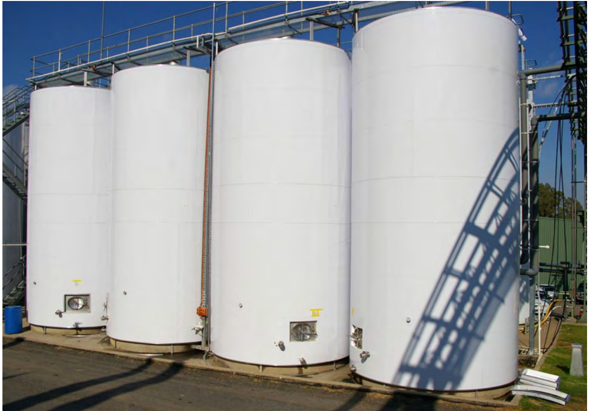
Figure 10. Example of insulated wine tank to control temperature of the contents.
